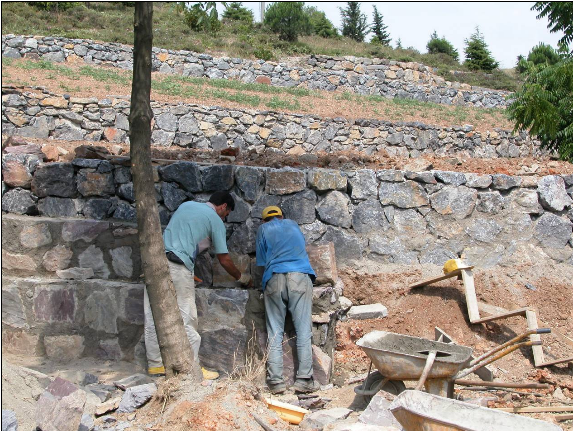
Construction work in the amphitheatre, 2006
